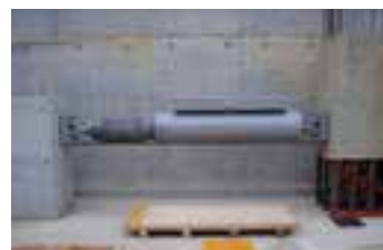
Seismic isolator (oil damper)
