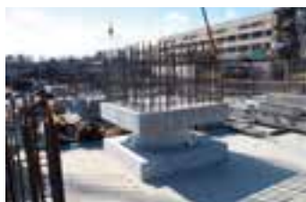
Seismic isolator (elastic sliding bearing)
