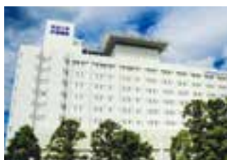
KEYAKI Building exteriors ①
