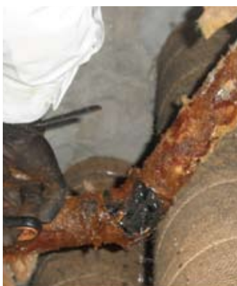
● 給水管破損
